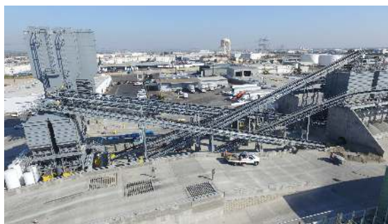
Above: National Ready Mixed Concrete LA
