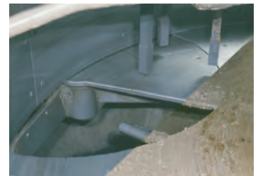
High Pressure Cleaning
